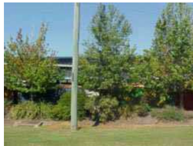
Before: Limited surveillance of rear of building due to landscaping and lack of maintenance
