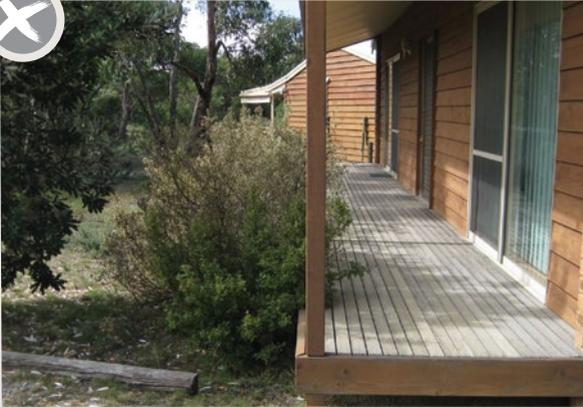
*Trees and shrubs abutting the home increase the effects of direct flame contact and radiant heat.*
