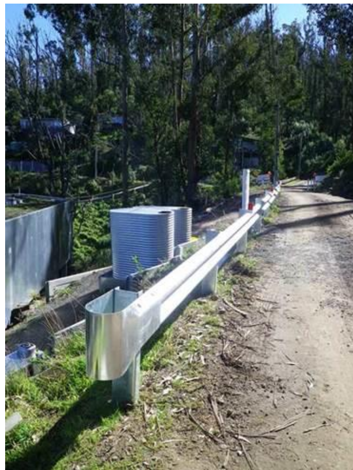
New guardrails throughout Wye River and Separation Creek
