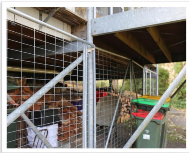
Figure 31 Heavy fuel stored under a house
