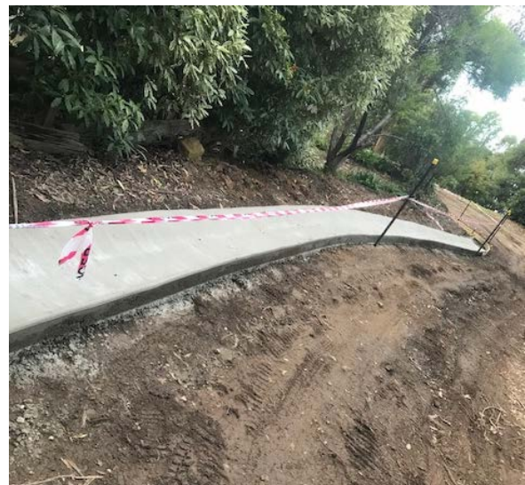
Slashers Bypass kerb works
