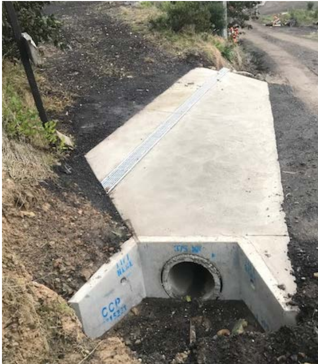
Driveway culvert – Bass Ave
