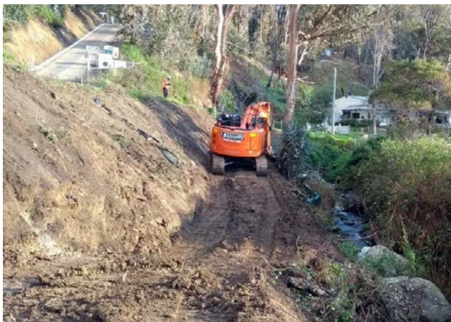
Stanway Drive works
