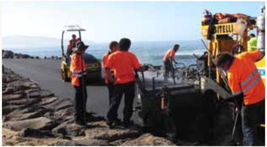
Above: Asphaltting the road on the Apollo Bay breakwater wall.
