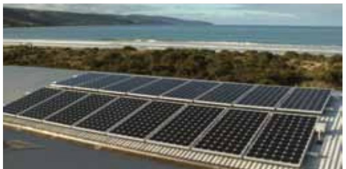
ABOVE: Apollo Bay Visitor Information Centre solar power system
