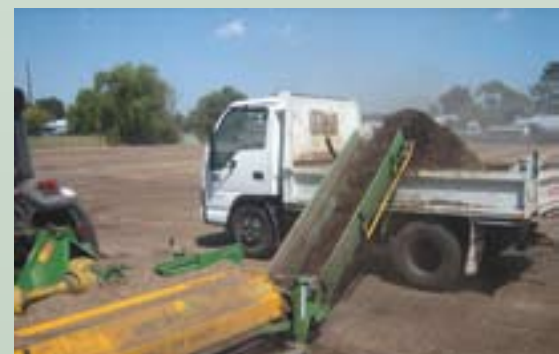
Redevelopment of the Hockey Fields at Central Reserve, Colac
