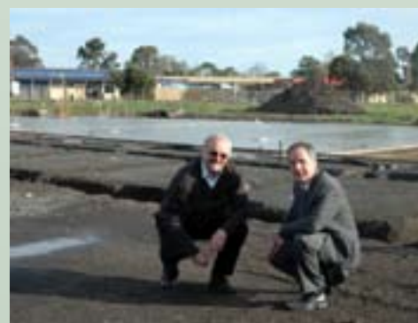
Mayor Brian Crook (left) and Richard Cooper (right), Principal of Colac Secondary School at the pouring of the slab for the Joint Use Library
