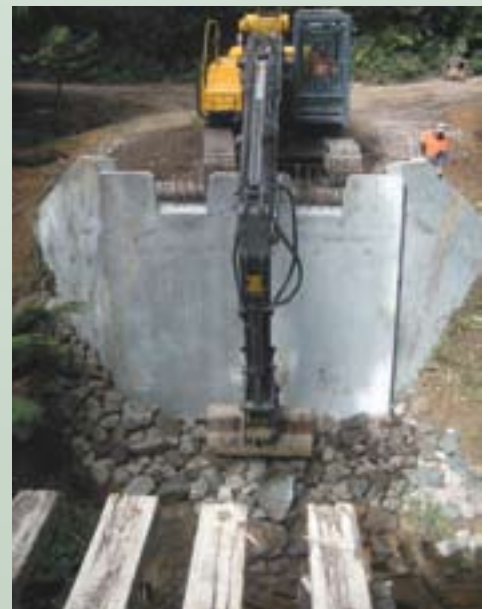
Binns Road bridge under construction at Aire River
