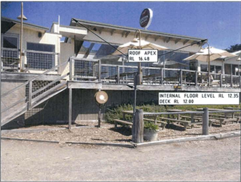
PHOTO 3 HOTEL ROOF DETAIL & DECK / FLOOR LEVELS
