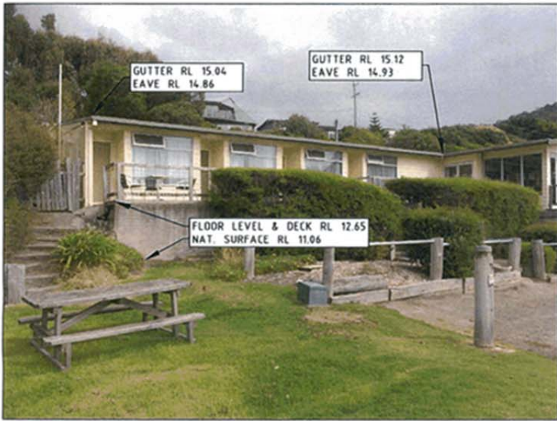
PHOTO 1 MOTEL - FRONT ROOF DETAIL
