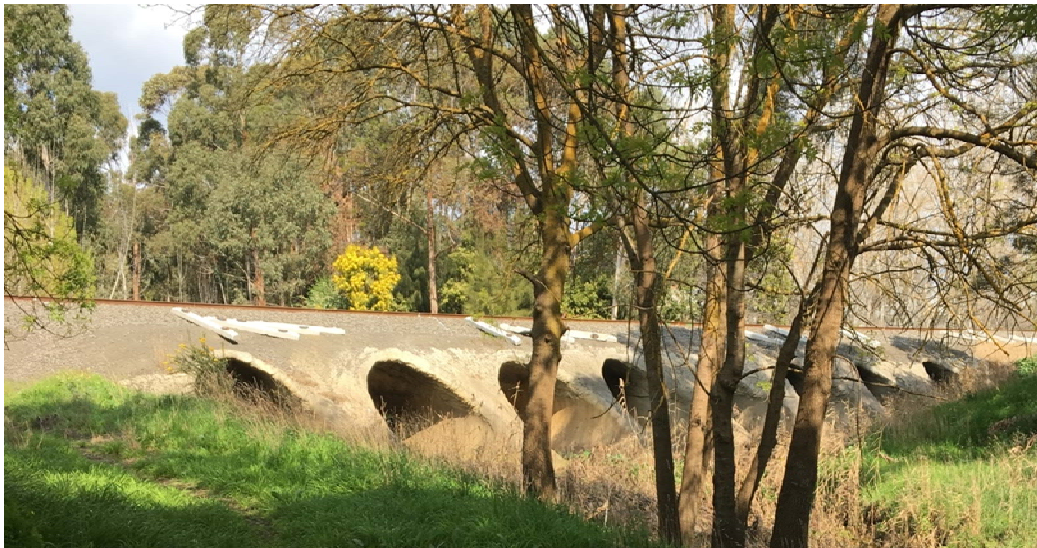
Under Railway culverts discharging into Barongarook Creek, north of Wallace Street
