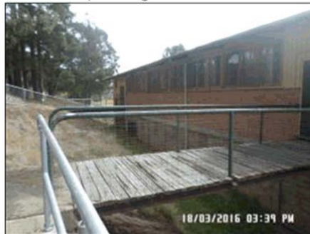
Ramp entry to first floor
