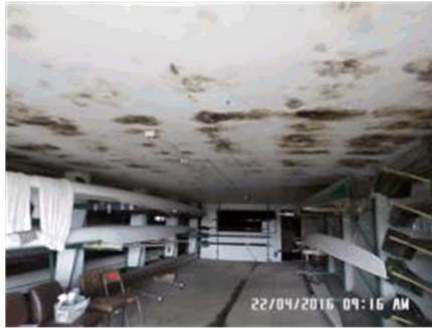
Damaged Roof Ground Floor
