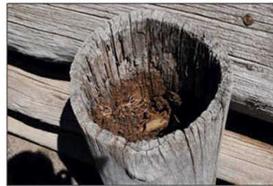
Retaining wall located behind the main pavilion, and one of the retaining wall posts showing the effects of termite infestation
