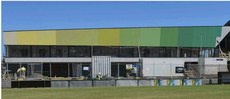
Central Reserve club rooms under construction
